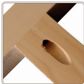
POCKET SCREW JOINT
